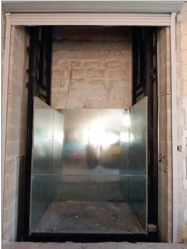
Il-Goods Lift installat.
