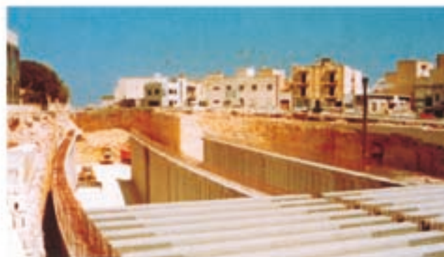
Msida multi-level intersection
