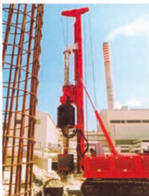
Piling works for Enemalta, gas turbine foundations
