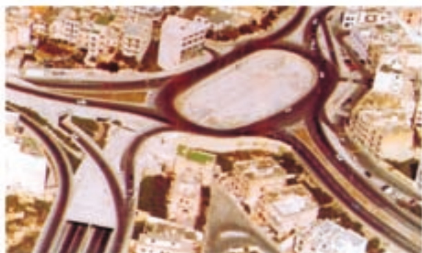
Msida multi-level intersection
