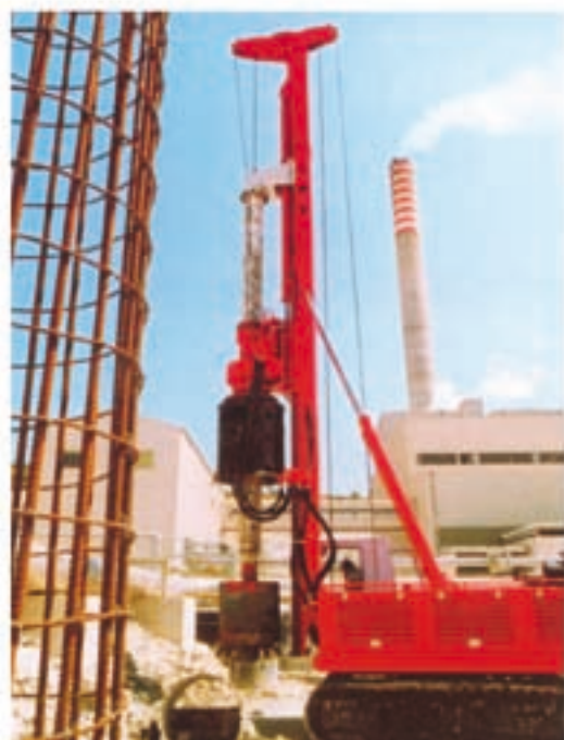
Piling works for Enemalta, gas turbine foundations
