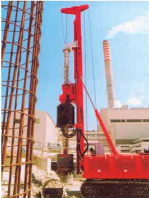
Piling works for Enemalta, gas turbine foundations
