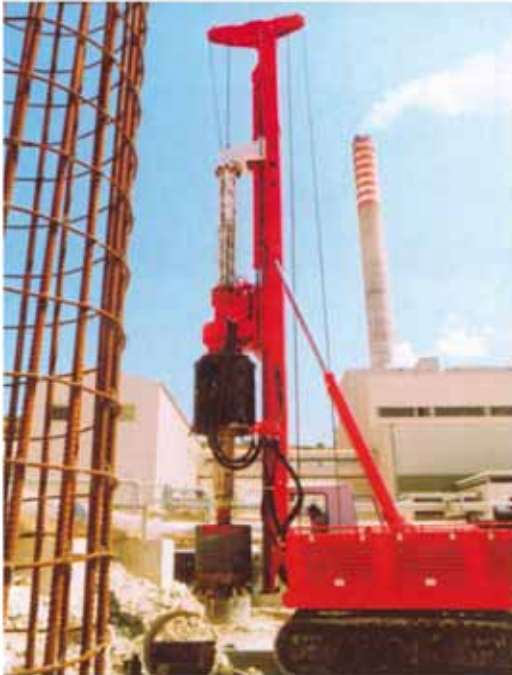
Piling works for Enemalta, gas turbine foundations
