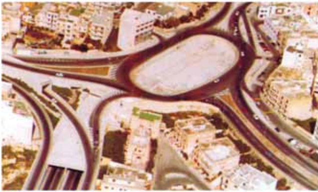
Msida multi-level intersection
