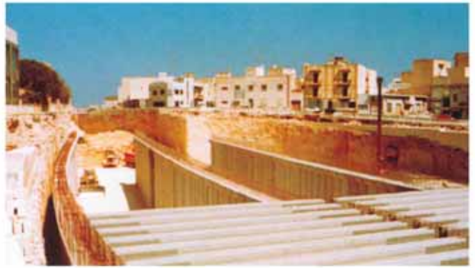
Msida multi-level intersection
