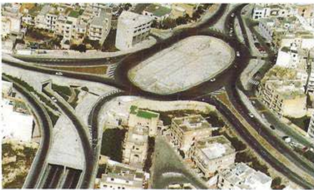
Msida multi-level intersection
