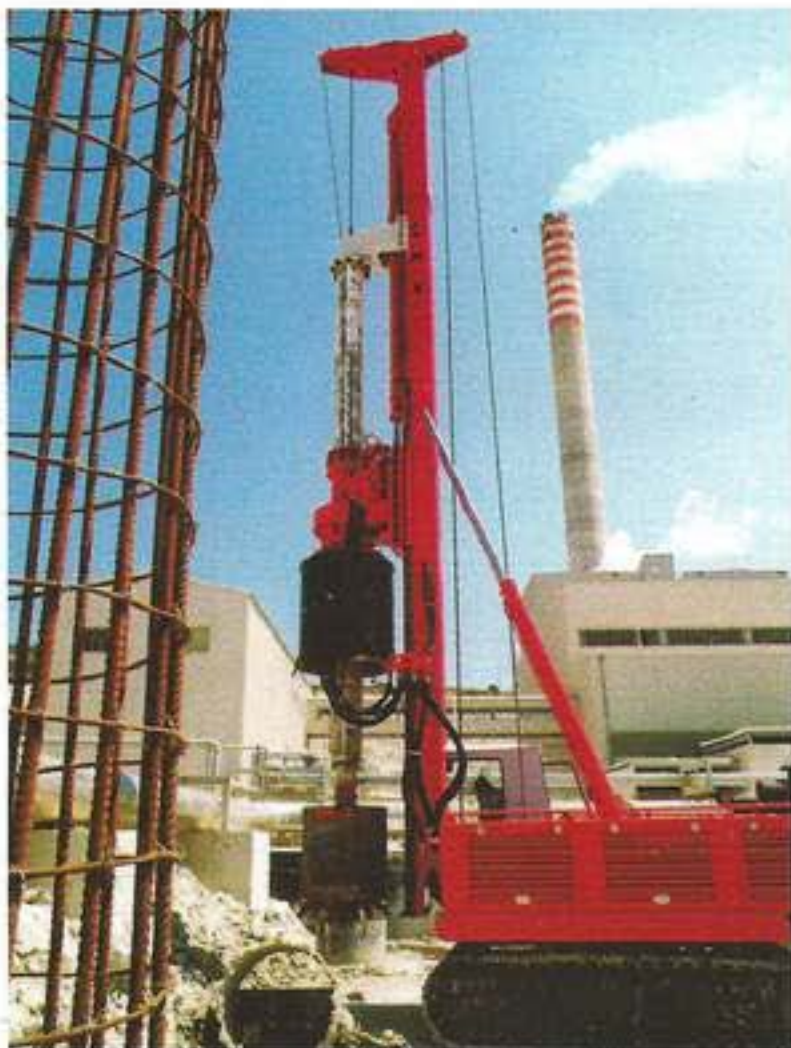
Piling works for Enemalta, gas turbine foundations
