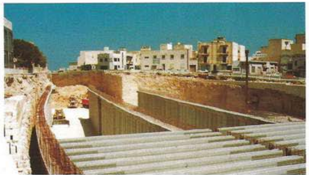
Msida multi-level intersection
