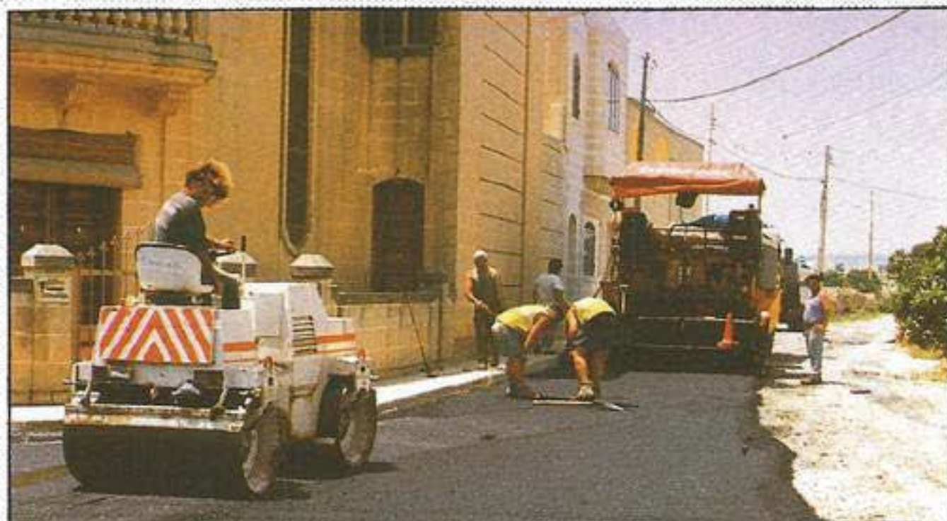
ROAD SURFACING WORKS IN PROGRESS AT KIRKOP - MALTA
