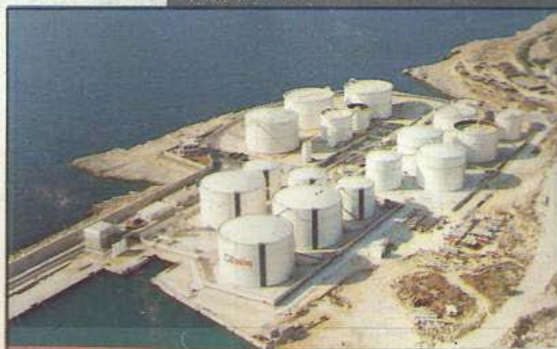
OILTANKING TERMINAL PHASES I & II
