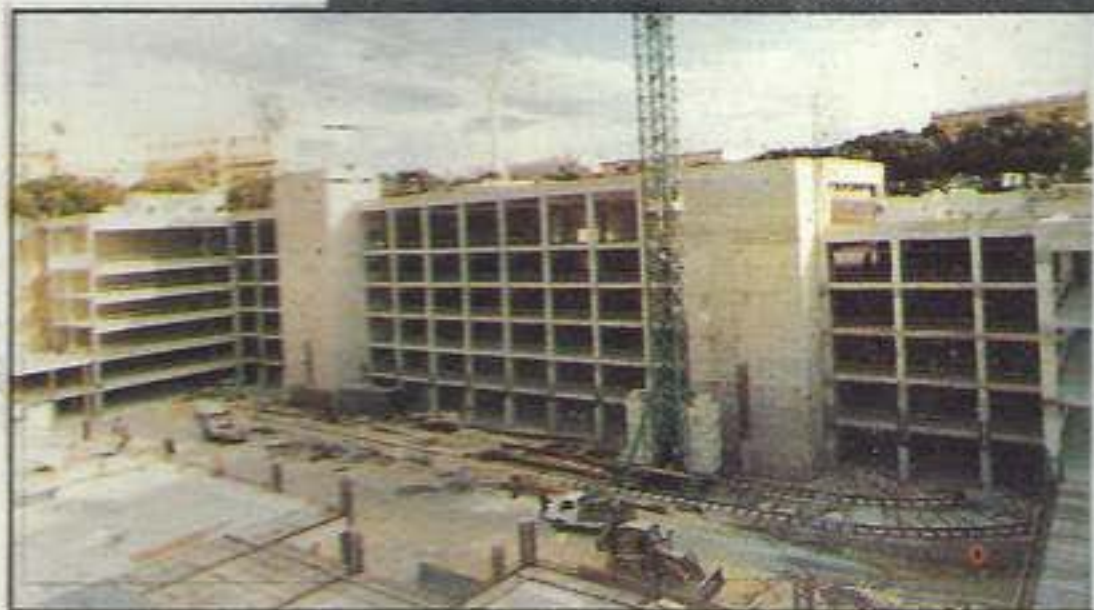
CONSTRUCTION OF CAR PARK - FLORIANA
