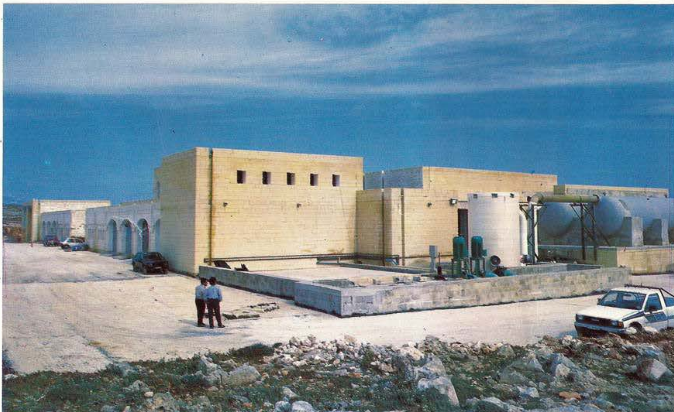
REVERSE OSMOSIS PLANT - PEMBROKE
